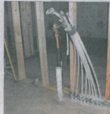
The Eco-Village home includes an Uponor radiant heating and cooling system in the floors. The community won't consume more energy than it produces.
