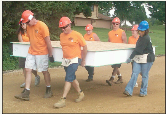
Volunteers from Andersen Corporation and a future eco-village home owner carry a Structural Insulating Panel (SIP) wall. Photo credit: Andersen Corporation.
