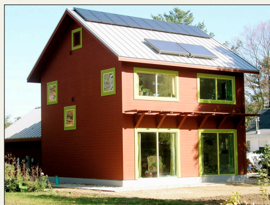
With special insulation and triple-paned windows, Sonya Newenhouse’s 970-square-foot NewenHouse prototype in Viroqua is Passive House Certified. Photo by Martin Jenich.
