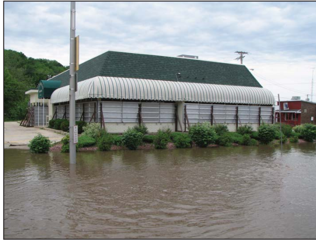
A Darlington business with flood shields installed shown during a 1998 flood. Photo: Phil Riseeuw, Darlington
